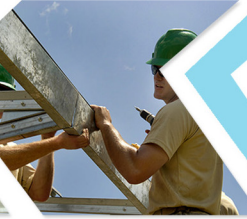
钢构搭建 Setting up
